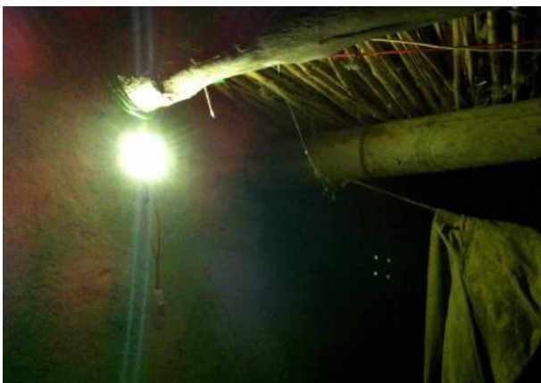
Figure 4.26: Micro-grid electricity connection for each household. (Source: www.meragaopower.com )
