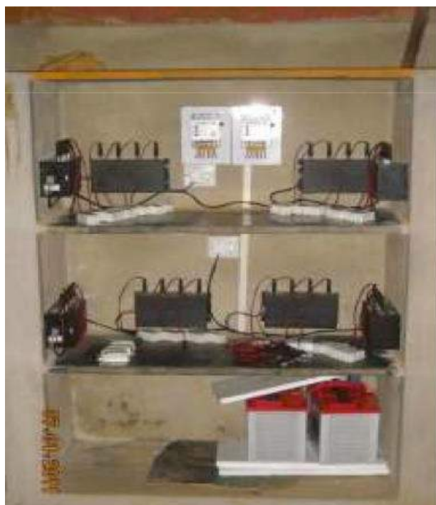
Figure 4.21: Solar central charging station for detachable batteries. (Source: Selco)
