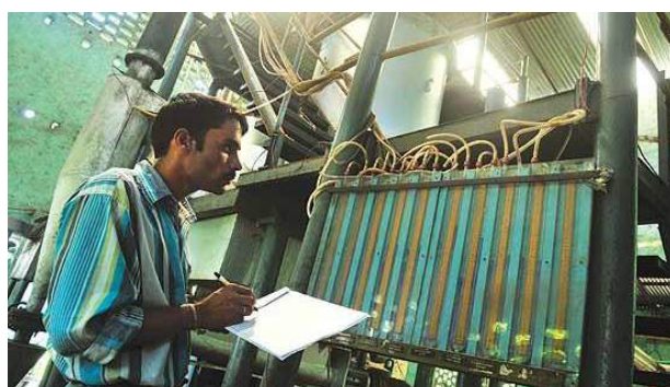
Figure 4.10: Local youths have been trained to operate and maintain the biomass power plant. (Source: Gopalan, 2011)
