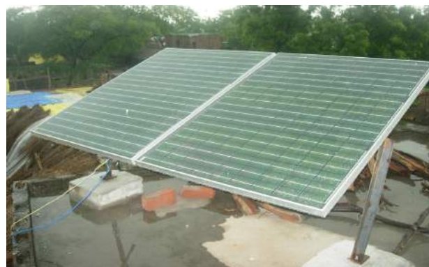
Figure 4.25: Solar Panels placed in the middle of the village. (Source: www.meragaopower.com )
