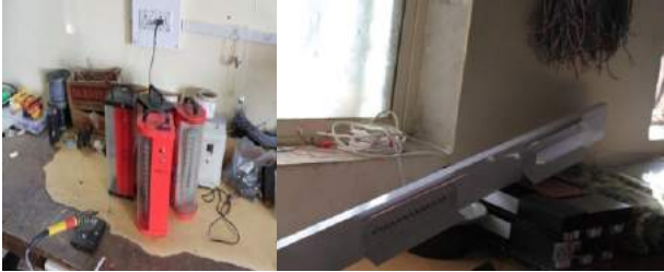
Figure 4.31: Solar lantern and PV based lighting system for school (Photo: Ruchi Jain)
