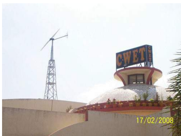
Figure 4.46: Small Wind installation at Centre for Wind Energy Technologies.
