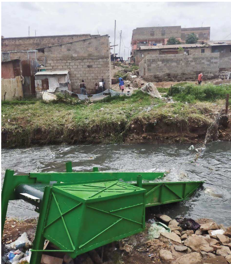
Image 9: Plastic capture system at the site.
