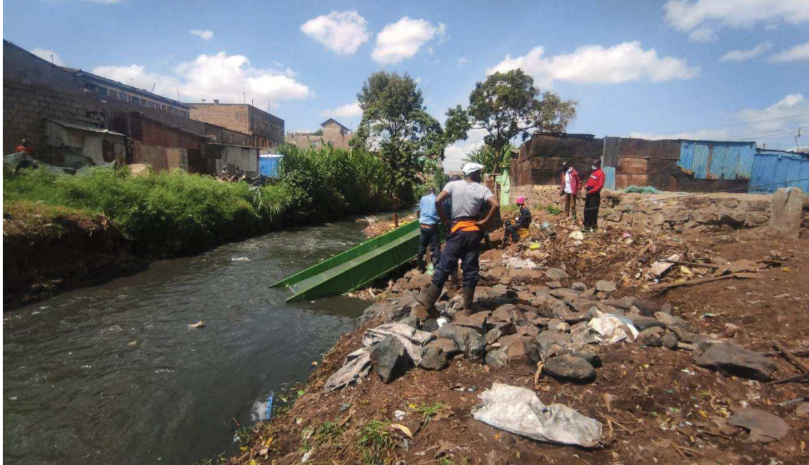
Image 7: Plastic capture system at the site.
