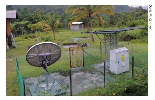
A village micro-grid system in Sabah, Malaysian Borneo. The system serves a community of 200 and provides household energy services, telecoms and satellite (dish shown), and water pumping for fishponds (seen at centre) and refrigeration. The supply includes microhydro and solar generation — one small panel is shown here and others are distributed on building rooftops.
