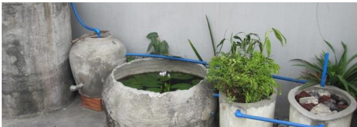
A simplified, low-cost wastewater treatment plant composed of biogas digester, anaerobic filter, gravel filter, planted gravel filter, and lotus pond designed for small spaces.
