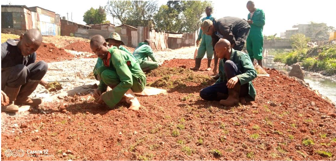
Image: Planting of Grass and rehabilitation of the illegal Dumpsites.
