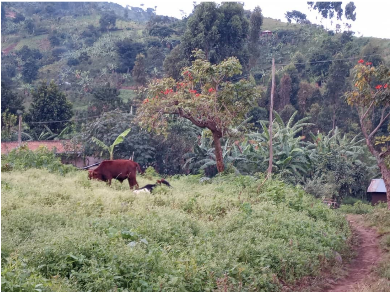
Transmission line to supply power to Mbata Primary School from the FEC
