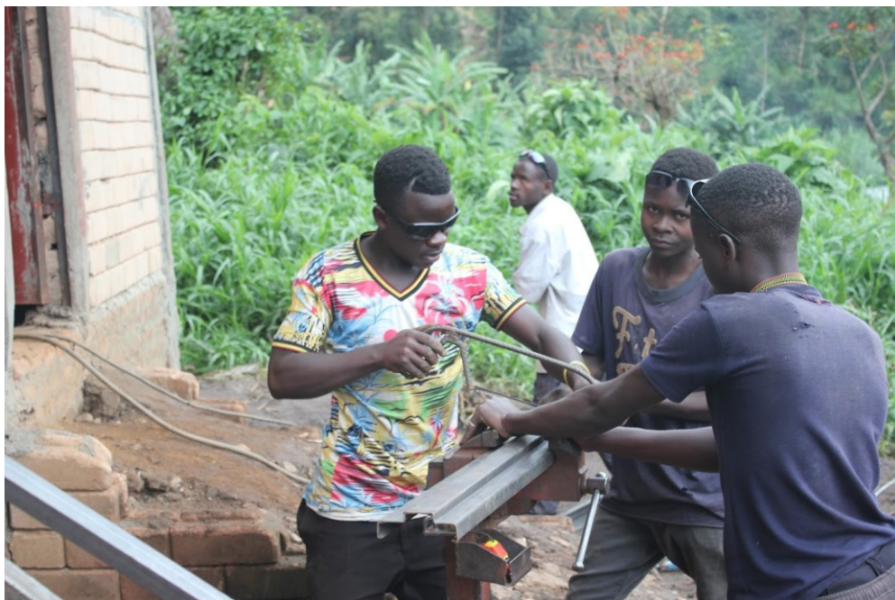
Metal fabrication and welding service in Mbata
