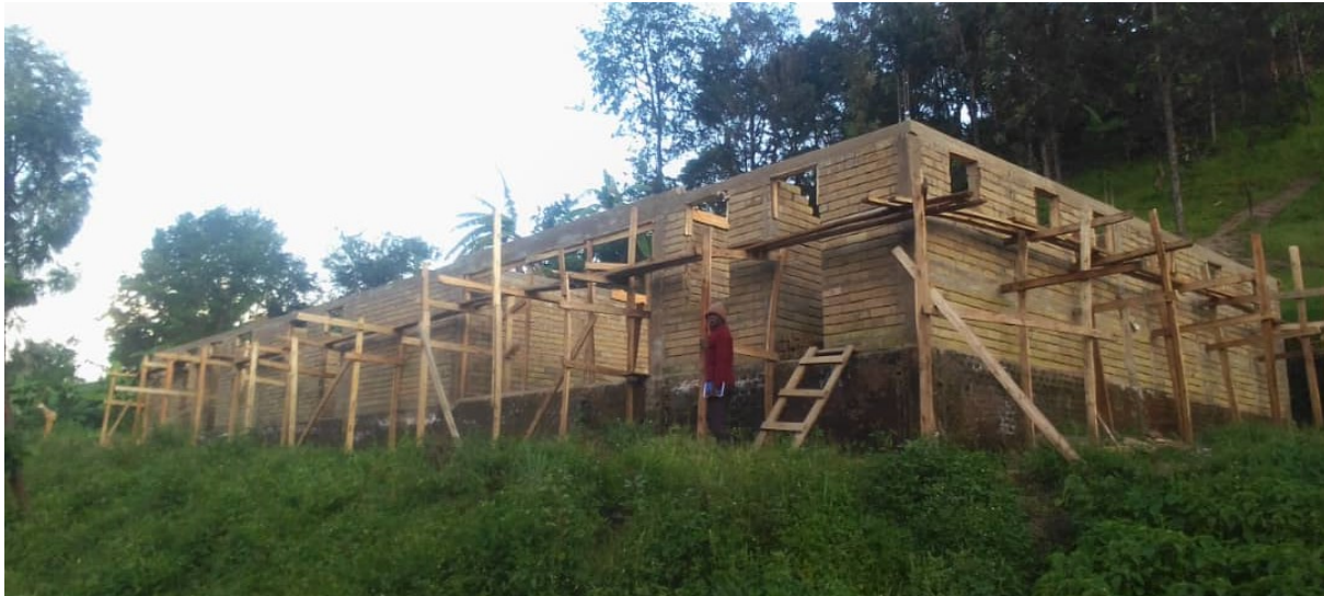
Mukorokumi FEC under construction
